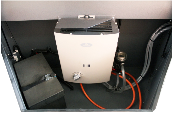
Instant on demand Hot Water Geyser with pressure pump.
